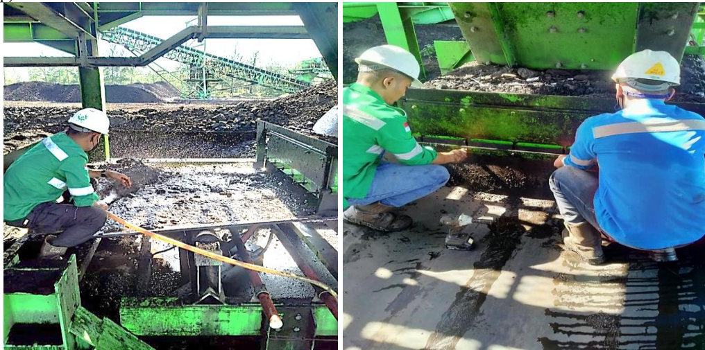
Gambar 2. Kegiatan perawatan belt conveyor
